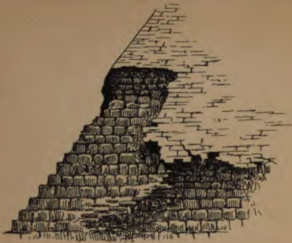
Masonry courses, backing stones, & casing stones of 2 nd Pyramid, near the upper part of S.E. angle. From Photograph.
