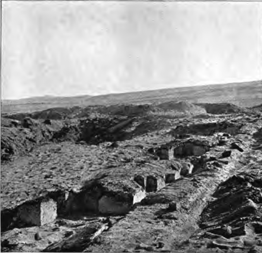
PANELLED BRICKWORK, WEST SIDE, LOOKING S.
