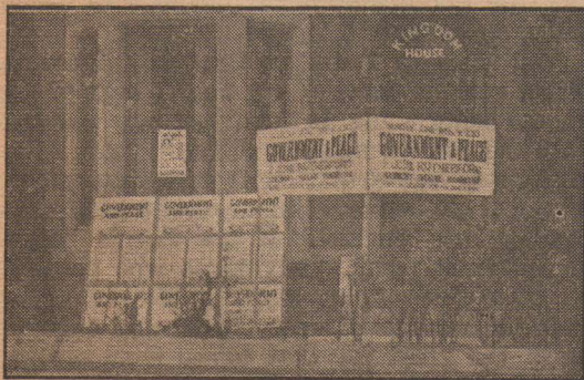
Kingdom House, Manchester, England
