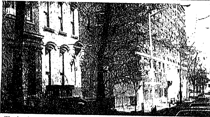
The headquarters of Jehovah's Witnesses, erected in 1949 at 124 Columbia Heights, was the first new building put up by the organization in Brooklyn Heights.
