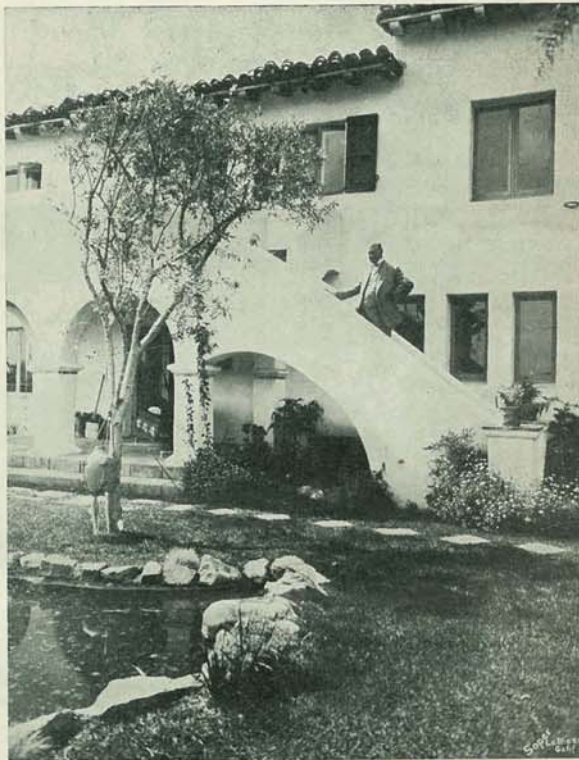
The Outside Stairs from the Patio to the Sun Parlor.
